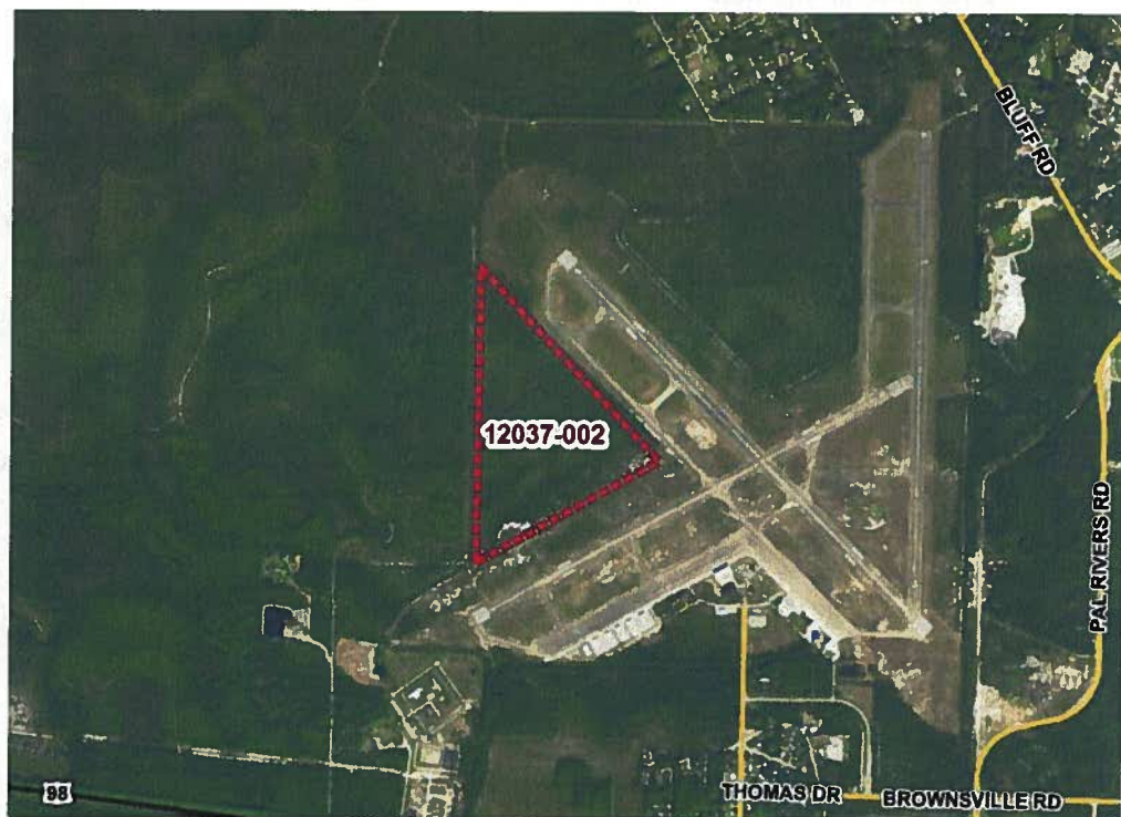
Figure 6.8: Franklin County Site 12037-002
